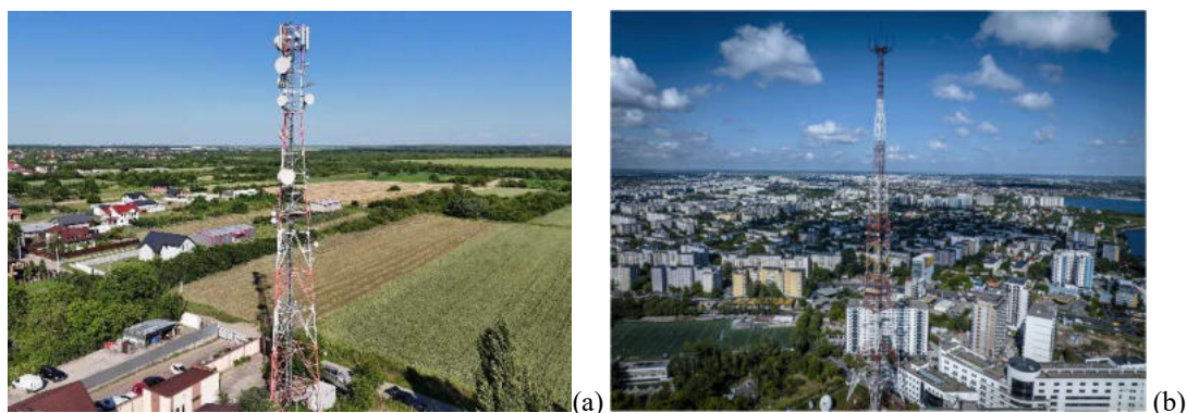
Figure 1. (a) The Afumați tower and (b) the Bucharest tower
