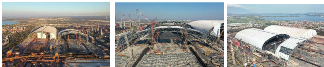
Figure 4. 3000t module lifting, translation, cladding phases
