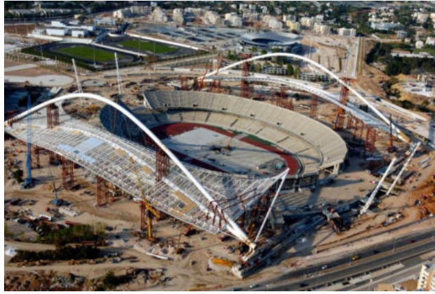
Figure 1. A view of the construction site a few months before the opening ceremony
