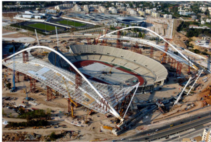
Figure 1. A phase of the construction site some months before the stating ceremony
