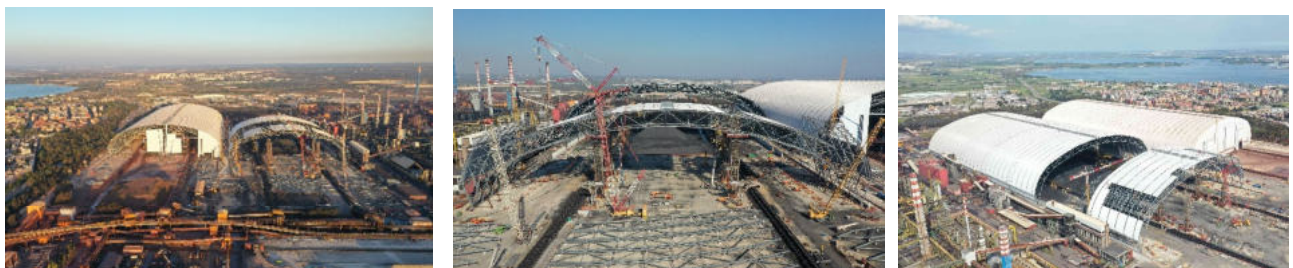
Figure 4. 3000t module lifting, translation, cladding phases
